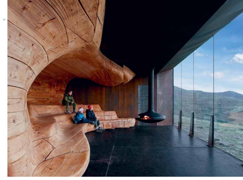
the manufacturing process," says Bjørgum. Snøhetta used 3-D CNC carving to design the grotto-wall-like wooden structure of the southern elevation. Traditional shipbuilders in Hardangerfjord, an area located just south of Bergen, created the wooden formation by layering numerous 10-square-inch pine beams, pinned simply together with pegs. The undulating ripples of the wood resemble the jagged topography of the Dovrefjell visitors to enjoy and savor panoramic views
