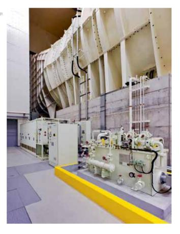
01 The exterior shell of the wind tunnel 02 The machine below the testing room is a weighing scale for vehicles 03 Precisely angled metal slats guide the air through in a steady motion
